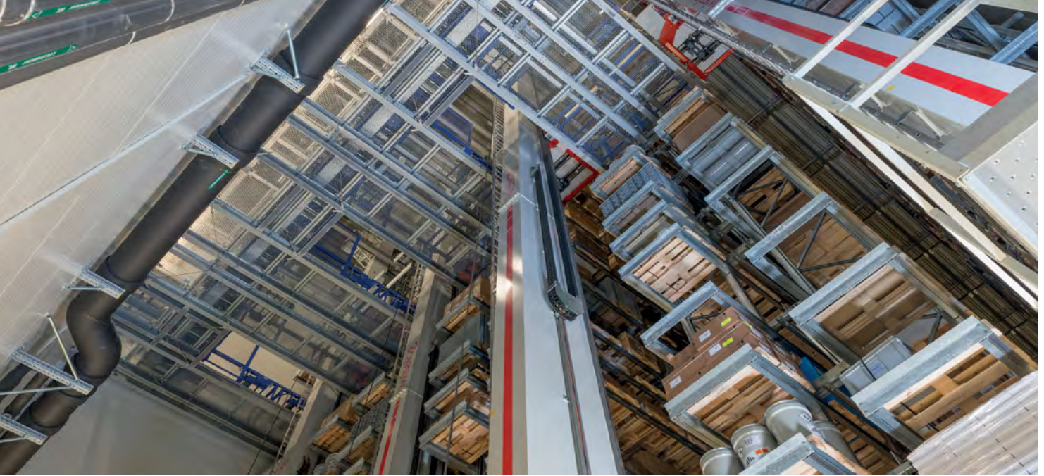
In the pharmaceutical industry, 100 percent product safety is essential. Swisslog ensures that the logistics system at Roche works reliably.
