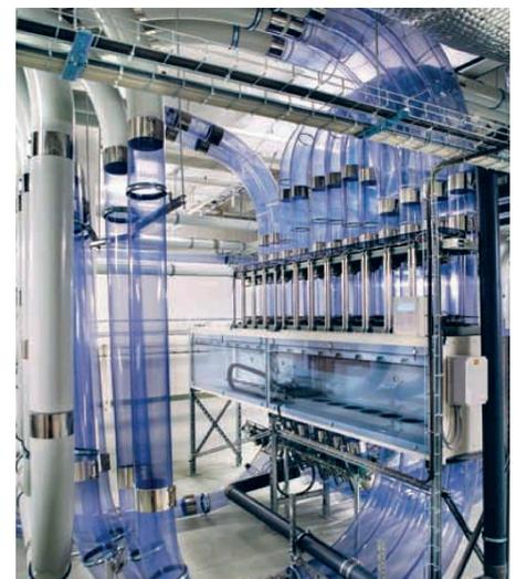
In this clinically sterile, un-manned special station, the carriers are automatically diverted to new tubes to continue on to their destination. In the bin with transparent sides, a carrier quickly transfers in the correct direction.
